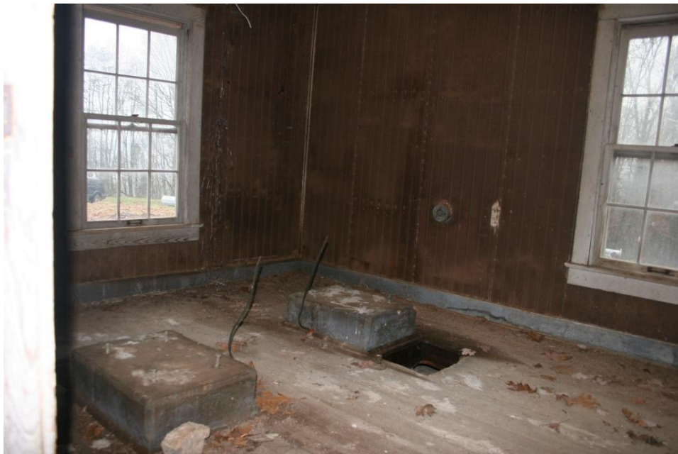
The location where the generator would have set on the two concreted foundations.
